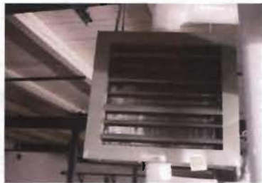
Hydronic Unit Heater Modine Model No. HSB193SB01SA (Year: 2018) Serial No. 43104417-2302 1/3 Hp; 115 V; 4.2 Amp Near Sed Basin No 5 South Side
