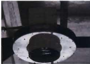
Chromalox Electric Unit Heater Main Floor Ceiling 277 Volt; 1 Phase VUH-1
