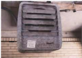
PFP - Sludge Building Heatflo Unit Heater - Electric Cat No. HLH-C-10-43-30-00 MFG Part No. 004-303380-503 10 KW; 480 V
