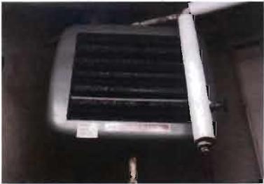
Modine Steam Unit Heater Model No. HS108S 01 Serial No. 0501039-5749 1/8 Hp; 115 V; 2.3 Amp Location: Hypo Room
