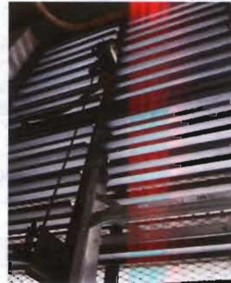
Siemens Actuated Louvers 7' X 4' Quantity: 2 Pump Station Basement
