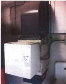
Exhaust Fan - EF-3 Location: Hypo Room Greenheck Model No. BSQ-70-4 Serial No. 06H026916 Belt: 3L-360
