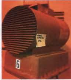
Electric Unit Heater - EUH-6 Marley Electric Heater Model No. W75041A Corrosion Resistent/Washdown MFG Code - L94 7.5 KW; 240 V; Single Phase Location: Pump Station
