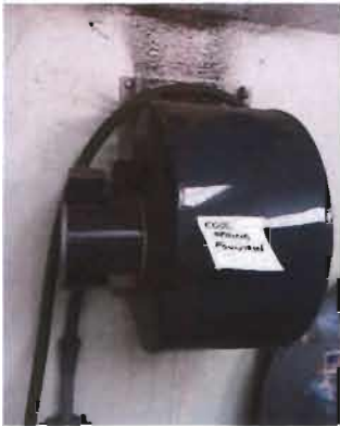
Blower Dayton Model No. 1TDU2 1/2 Hp; 115/230 V 1320 RPM; 1202 CFM Location: Fountain Pit near Park
