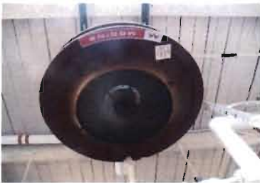
Modine Steam Unit Heater Model No. V139S 06 SerialNo. SP011996 Quantity: 2 Location: Locker Room/Sed Basin 8-10
