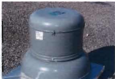
Cook Ventilator EF-6 Model No. 135ACE 135C15D S/N: 076SE49822-01/0003201 0.5 Hp; 2100 CFM; 115 V; 1 Phase Jan-13
