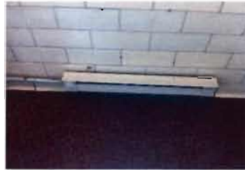
Electric Baseboard Heaters Quantity: 2 110 V; 15 Amp
