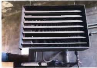
Trane Unit Heater Model No. UHSA126S6AAA Type: 136-109-01 Serial Number D83L03604 Location: Maintenance Shop above boilers
