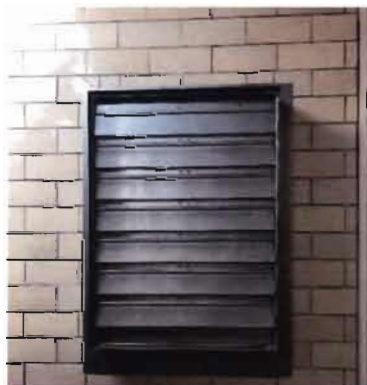
Two Gravity Louvers Located in Duct Room To Be Cleaned Annually
