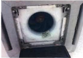
EMI Ductless Series Split Unit Model No. S1HG2000D12 Serial No. 1-12-F-6919-24 208/240 V; Single Phase Location: Control Room
