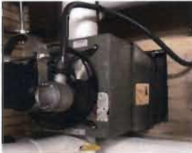
Carbon Room Modine Model HSB 33SB06SA 1/6 HP; 115 V; 2.1 Amp S/N: 18101819-5024
