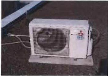
BMP - Rooftop Units Mitsubishi R410A, Mr. Slim Split Unit Matches to Meter Shop Office Model MUZ-09NA 208/230 V; 1 Phase S/N: 6003328
