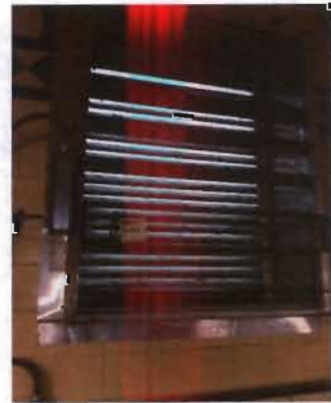
Eight (8) Actuated Louvers - Various Sizes Belimo Model FSNF24US Spring Return Actuator 70 in-lbs, 15S, 24 VAC Location: Throughout Membrane Area
