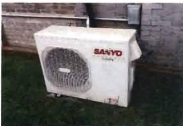
Sanyo Split Unit Model No. CH0971 Serial No. 0105212 85221344550000 115 V, Single Phase Plant Supv Office
