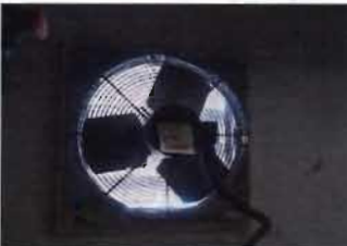
Lime Silo - Lower Dayton Fan Model 2C713B 1550 RPM; 1/20 Hp; 115 V; 1.8 Amp
