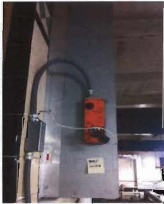
Eight (8) Actuated Louvers - Various Sizes Belimo Model FSNF24US Spring Return Actuator 70 in-lbs, 15S, 24 VAC Location: Throughout Membrane Area
