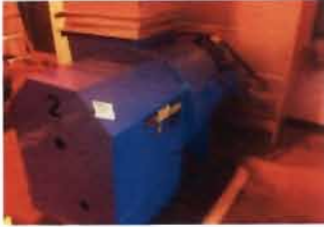
Exhaust Fan - EF-2 Twin City Fan and Blower Size 182; Type: BCV ARR. 10; Serial No. 7818612 With Actuated Damper Belt: 4L-330
