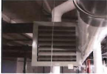
Hydronic Unit Heater Modine Model No. HSB193SB01SA (Year: 2018) Serial No. 43104417-2301 1/3 Hp; 115 V; 4.2 Amp Near Sed Basin No 3 South Side
