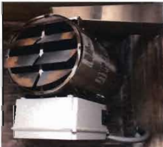
Screen House - Marley Electric Unit Heater Model No. QWD05212BT000 240 V; 5 KW; 1 Phase; 22.6Amps
