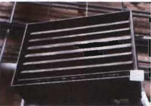
Steam Unit Heater Trane Model UHSA 12658AAAE Type 136-109-01 S/N: D83M03888 Location: Boiler Room
